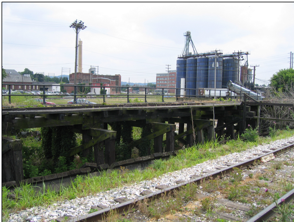
Photo 6: View of abandoned timber trestle between mainline and West Branch.
