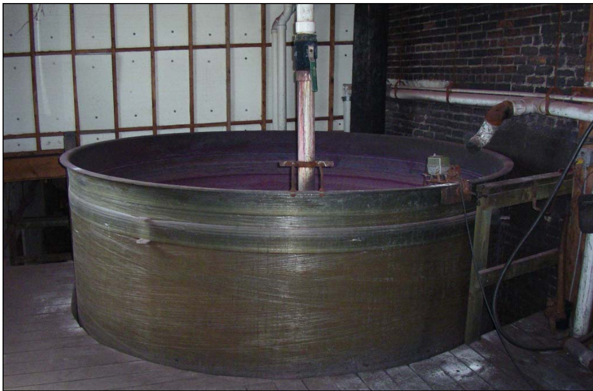
Photo H: One of three wastewater treatment tanks (Keystone Color Works)
