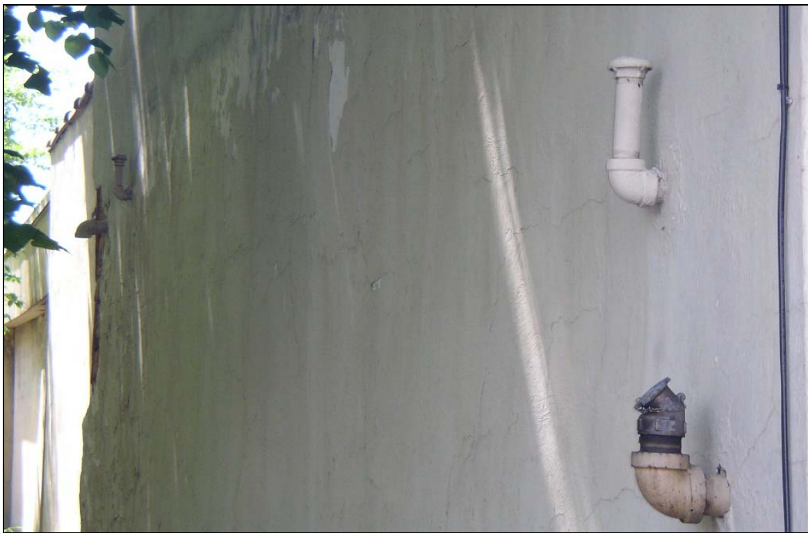
Photo B: Storage tank vent and fill pipes for unknown tank (left) and two 275-gallon heating oil ASTs (146-150 North Beaver Street)
