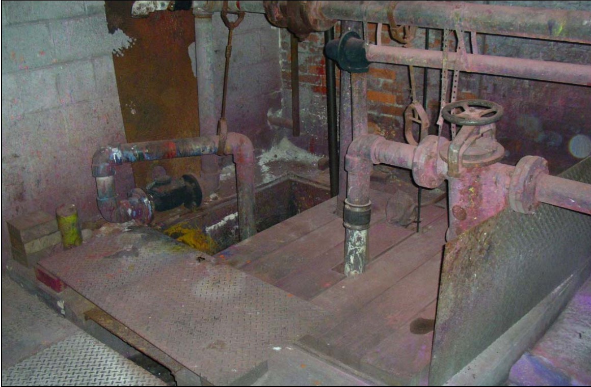
Photo G: Concrete wastewater holding pit on ground floor (Keystone Color Works)
