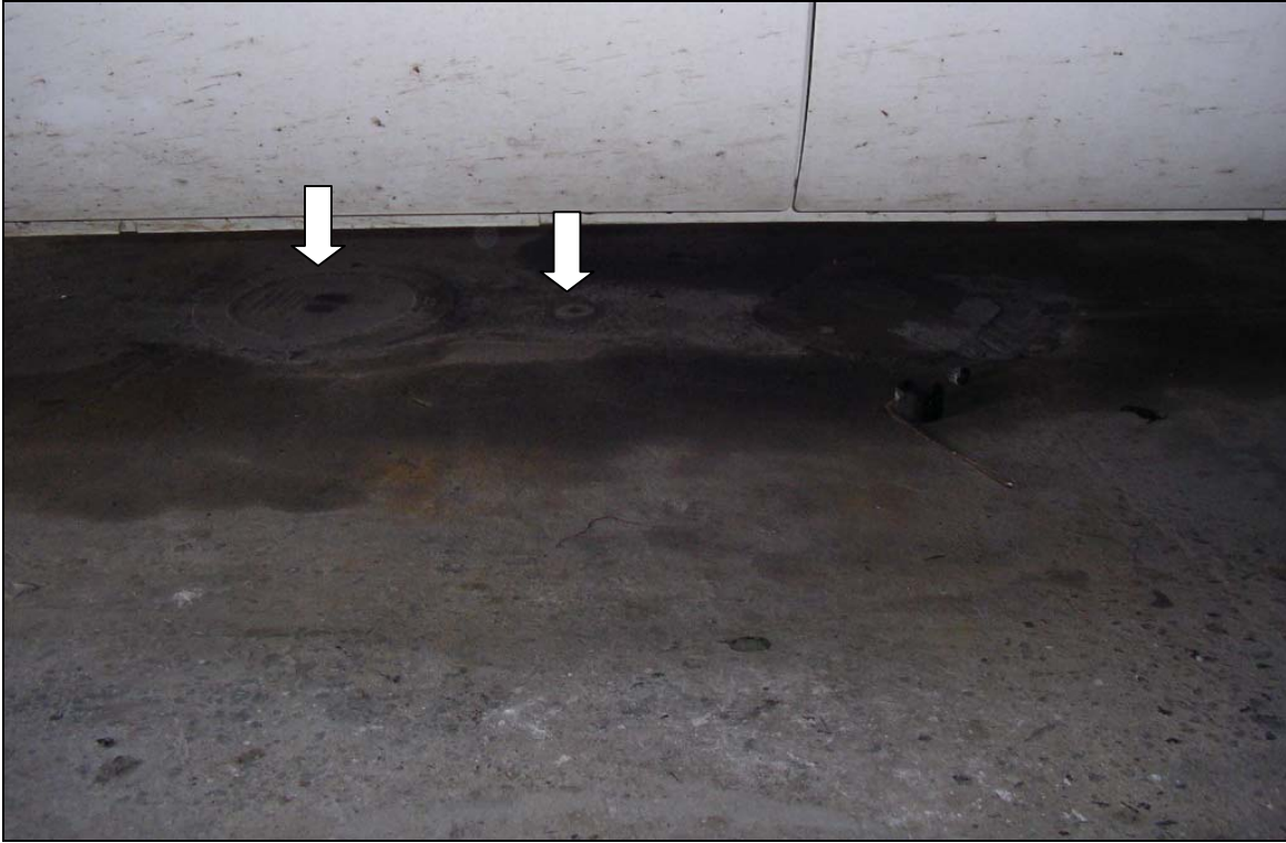
Photo K: Large (left) and small (right) floor drain caps at Weaver's Auto Body (208-236 North Beaver Street)
