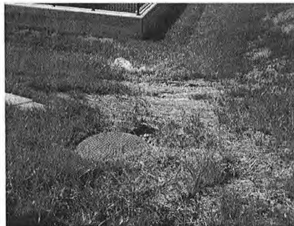
Erosion in slope above retaining wall.
