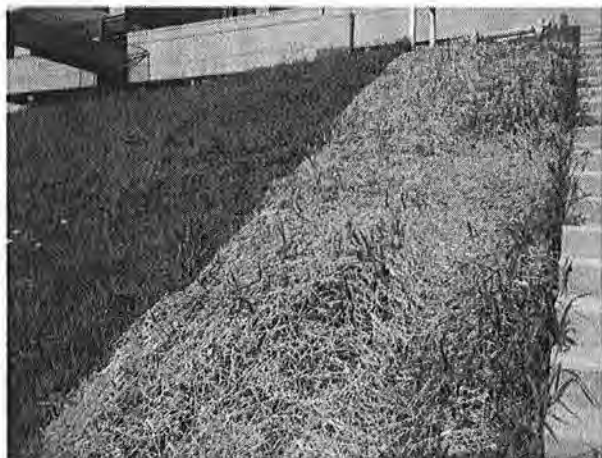
Erosion control matting along steps – grass pushing up matting
