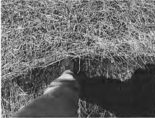
Matting in emergency spillway
