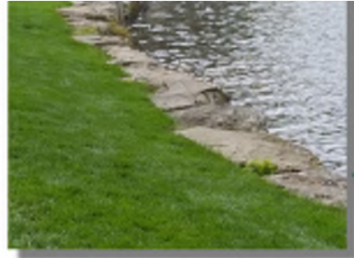
Riprap at water's edge
