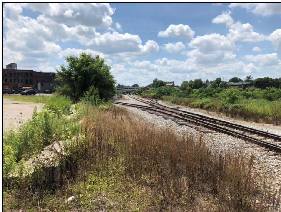
Westerly view of railroad trails boarding SP 3 (SP 3 to the left)
