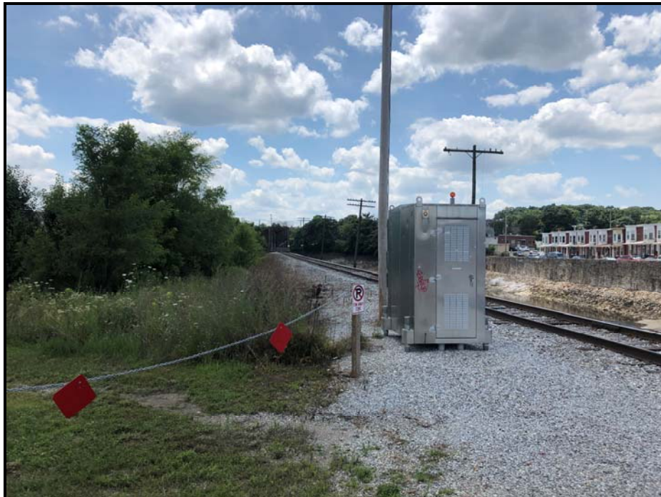
Westerly view of railroad line bordering SP 1 (SP 1 to the left)
