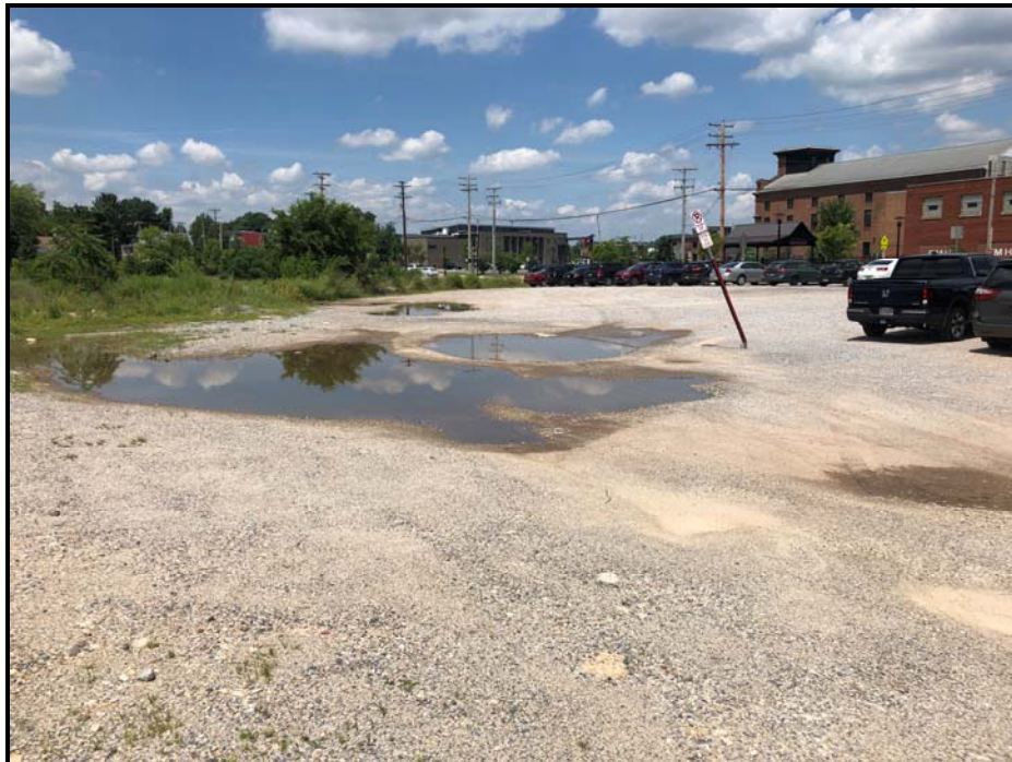
Pounding located on SP 3
