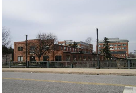
Market Street Bridge—View nw toward west bank, offices old and new
