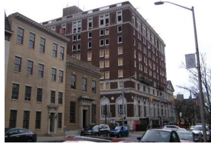
Yorktowne Hotel redevelopment project—Hilton Tapestry Collection—E Market St
