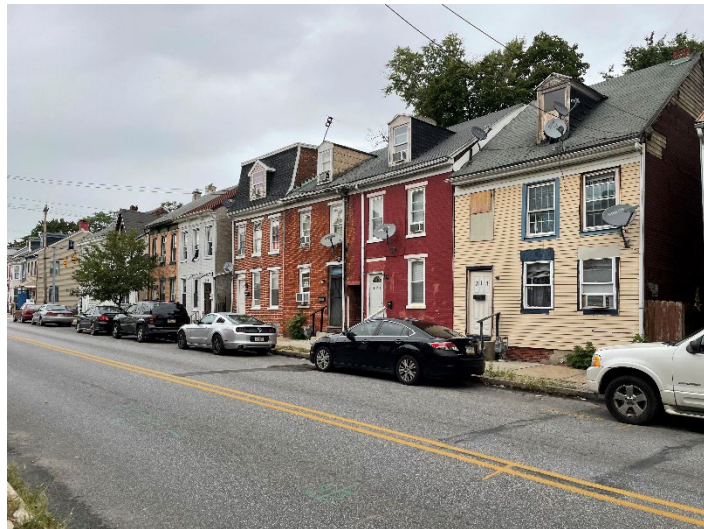
Figure 1 – 300 Block of South Penn Street
