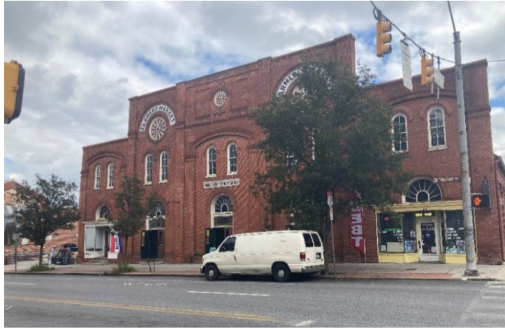
Figure 54 – Existing exterior of Penn Market
