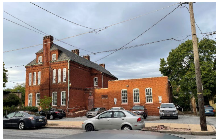
Figure 33 – Existing exterior of the Princess Street Center
