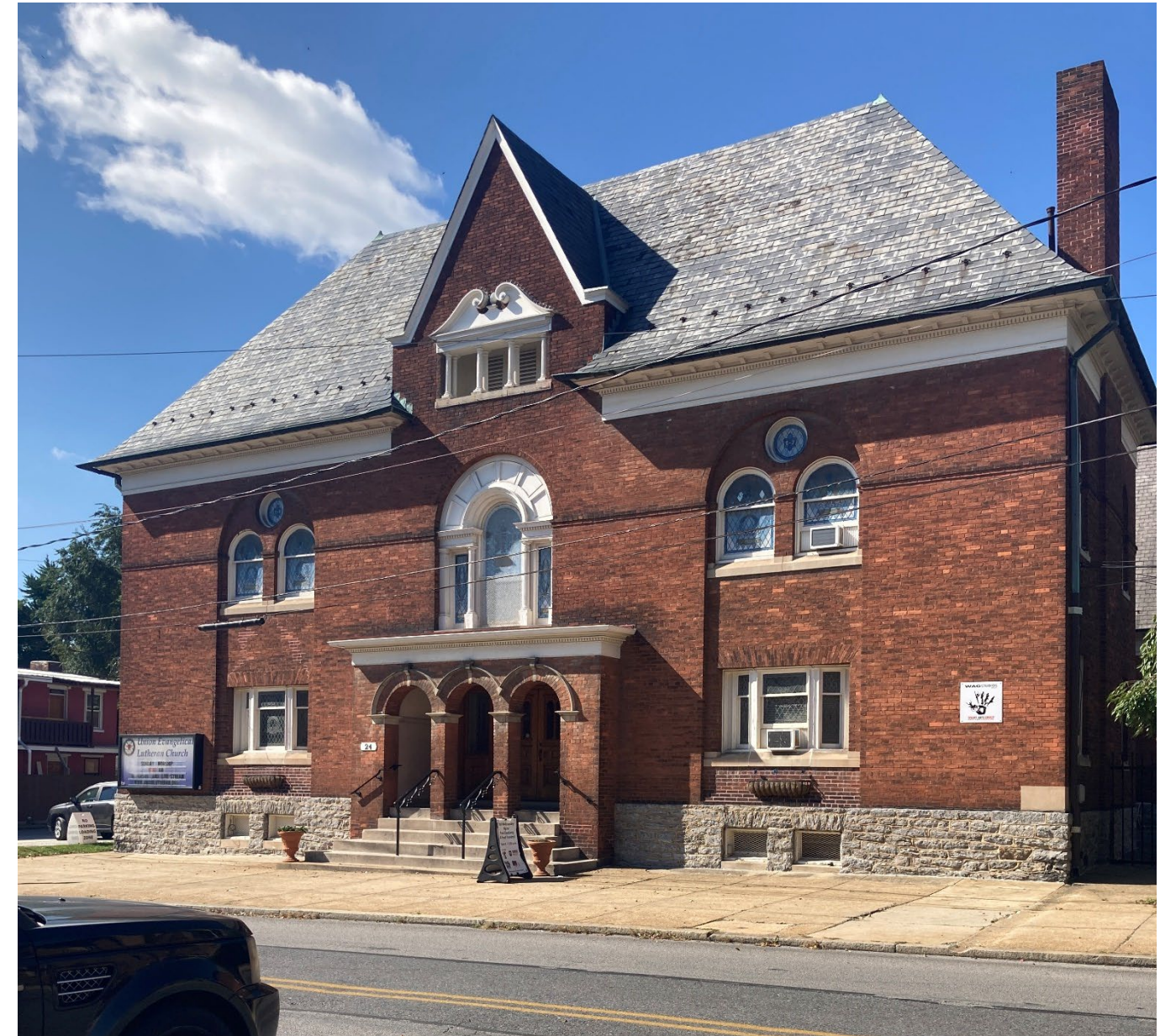
Figure 53 – Existing exterior of Union Lutheran Church on South Penn Street
