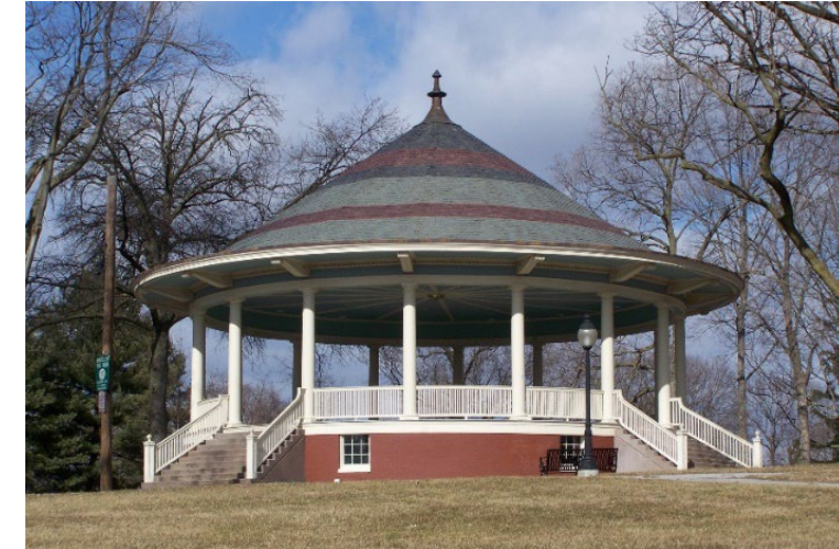
Figure 30 – Existing Farquhar Park pavilion
