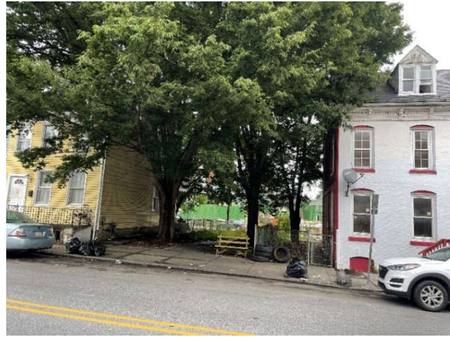
Figure 20 – Existing Thackston Connection
