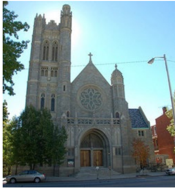
Figure 52 – Existing exterior of Union Lutheran Church on West Market Street ( www.unionlutheran.org )
