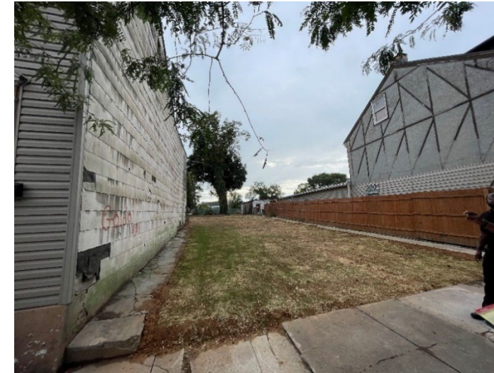
Figure 22- Existing Hope Street Connection
